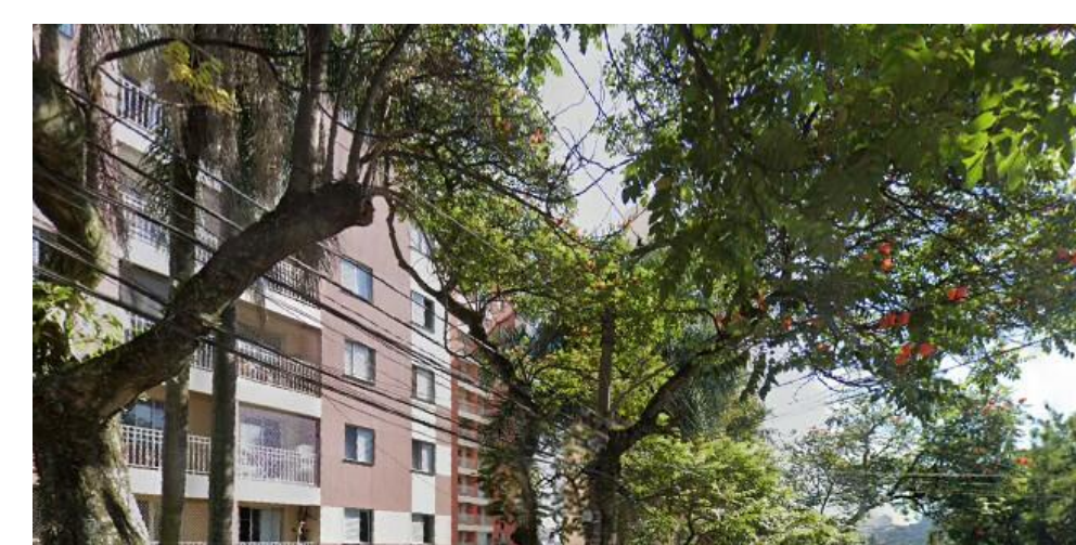
Fig. 1: Image from Google Street View with trees in contact with electrical wires.
